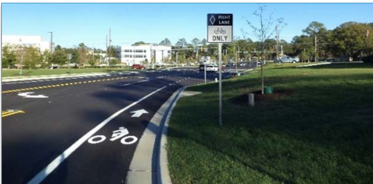
Figure 9. Bicycle Lane on Gornto Road, Source: SGRC
