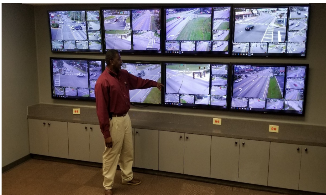
Figure 5. City of Valdosta Traffic Management Center. Source: Larry Ogden
